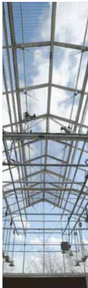
2 Lehman College's 69,000 sq. ft. New Science Facility, Phase I, showcases its strength in plant science teaching and research with high-tech sustainable laboratories, science learning centers and offices.
