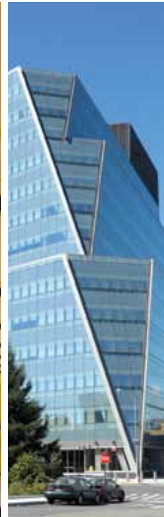
5 CUNY Law School moves to 2 Court Square, an environmentally green building in Long Island City with 260,000 sq. ft. of classrooms, library, law clinic, moot court, an auditorium and offices.
