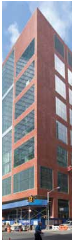
3 The new 390,000 sq. ft. Fiterman Hall at Borough of Manhattan Community College replaces the one lost on 9/11, with new classrooms, instructional and computer labs, an art gallery and café.
