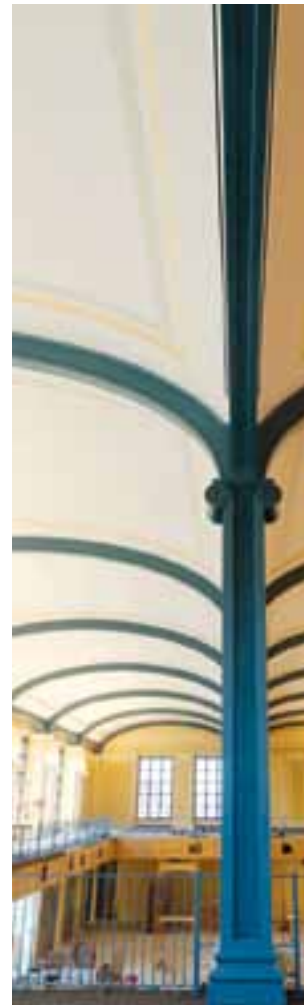
4 Bronx Community College's, 98,000 sq. ft. North Instructional Building and Library, provides classrooms, a library, a café, a two-story commons, study rooms and lounges.
