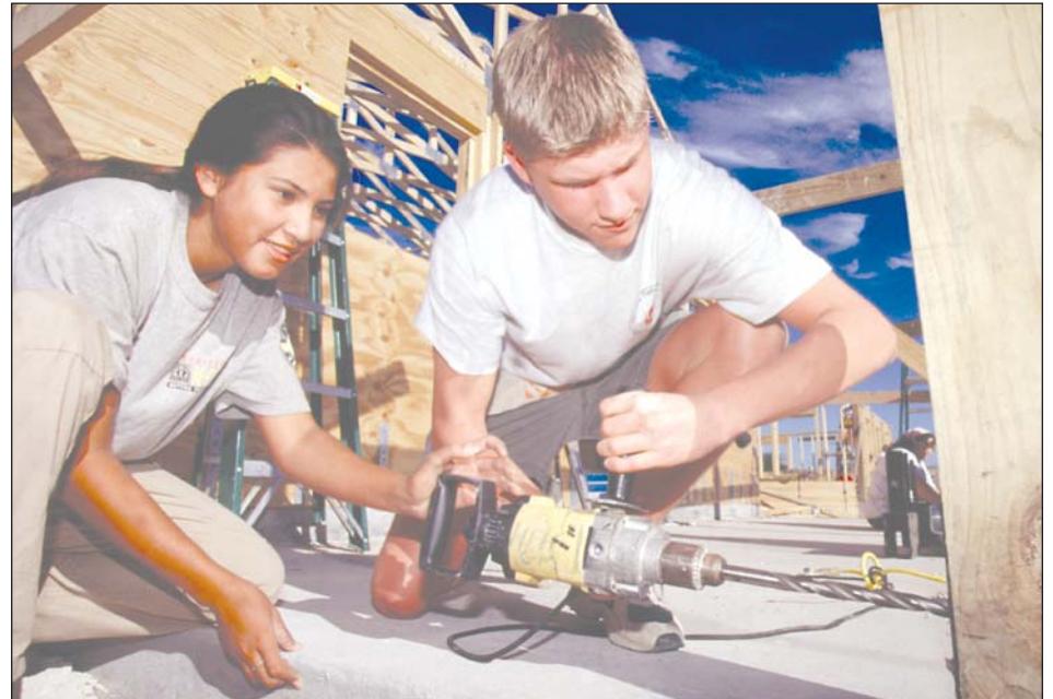
Drilling beams for support of new house.
